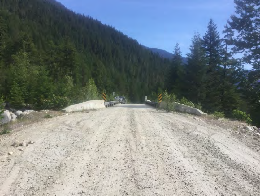
Approach from Right Bank when facing downstream
