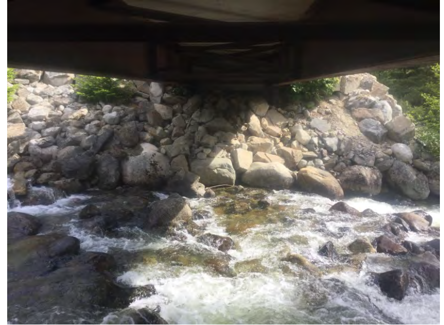
Left Bank Abutment when facing downstream
