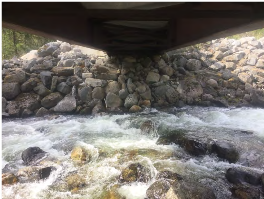
Right Bank Abutment when facing downstream
